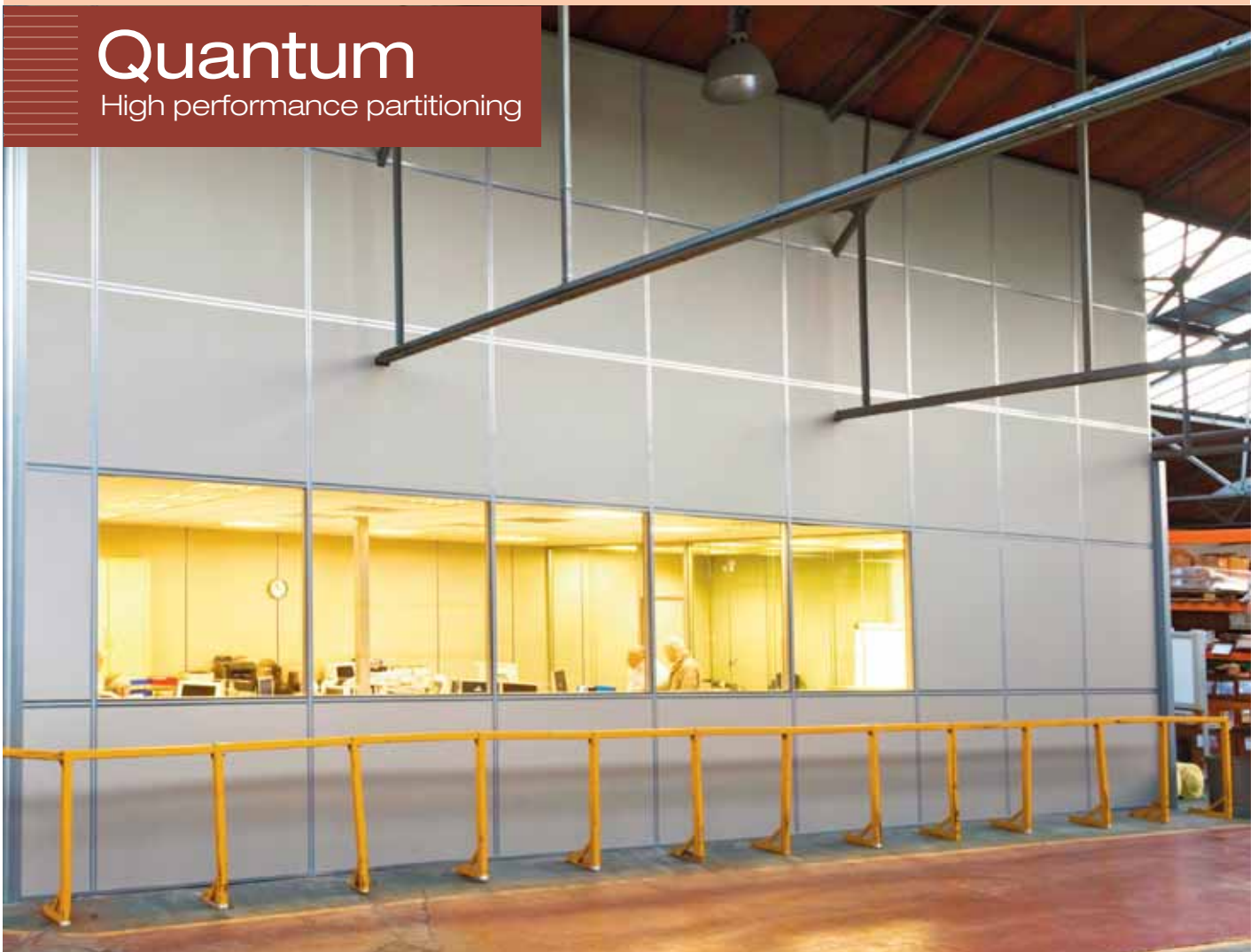
Quantum was assembled for protection in this 6 metre high light industrial area
